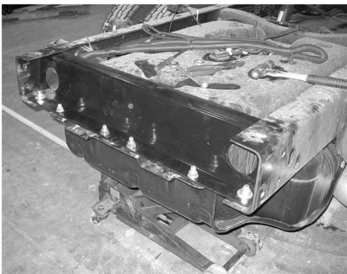
Bolt new crossmember onto fuel tank and truck frame.
