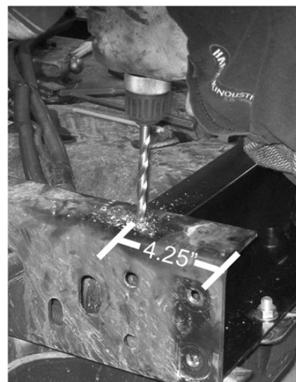
Drill new holes for top bolts (2).
